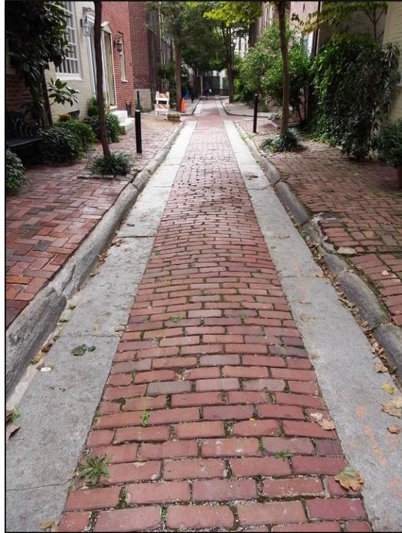
**Image 2:** Section of paving on South Jessup Street showing granite curbs, granite gutter stones, and brick pavers.
