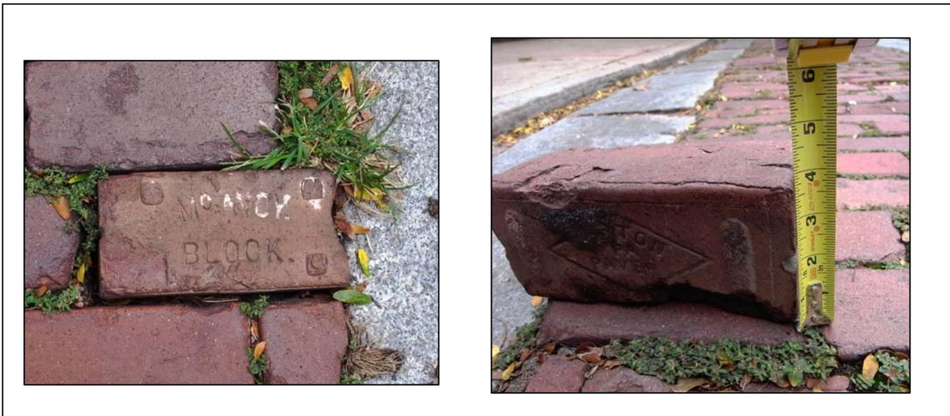
**Image 3:** Left: McAvoy Block vitrified brick paver Right: Patton Paver vitrified brick paver.
